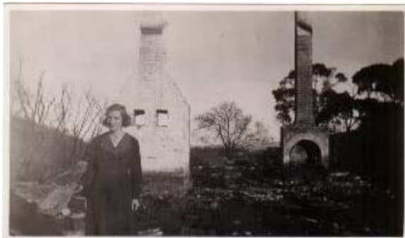
Dorothy Walker inspecting the ruins of the Parkinson's house at Steels Creek.
