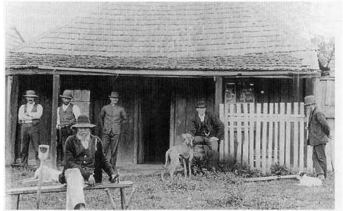
Yarra Flats Common School building – the chimney is at the right hand side
