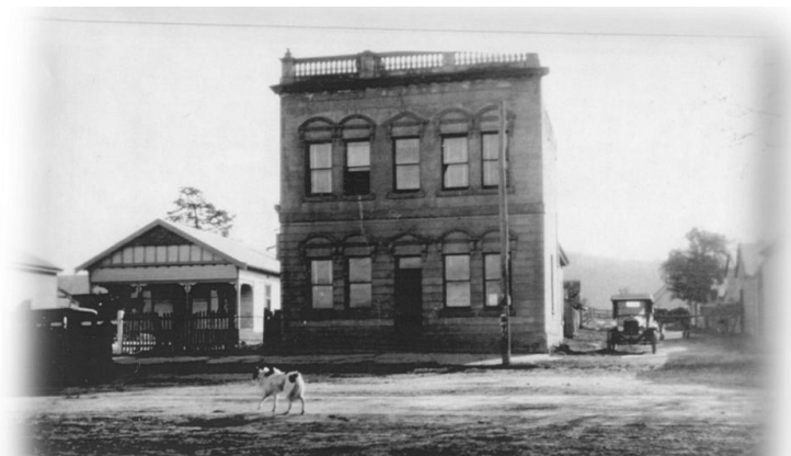
The building erected by William Herbert in 1890 as it was in the 1930s.
