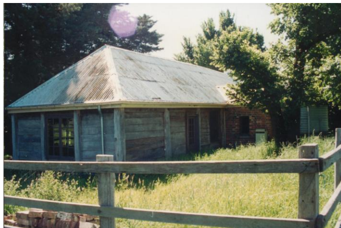
Elm Cottage showing the horizontal slab construction
